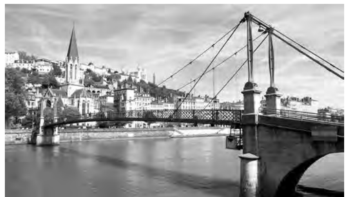
Lyon Passerelle St. Georges
